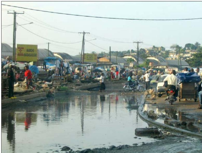
Photograph 3. Road Failure at Major Junction
