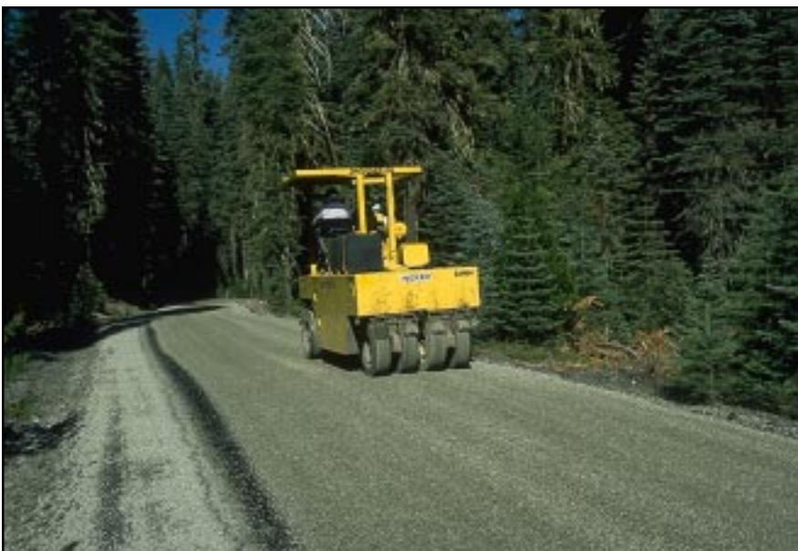
Photo 12.8 A chip seal road surface being compacted. A variety of surfacing materials can be used, depending on availability, cost, and performance.
