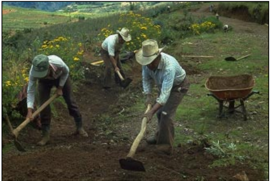
Photo 4.9 Perform road maintenance, either with equipment or by hand, to keep the roadway shaped and drainage structures functioning. Keep ditches clean but do not remove the layer of vegetative (grass) stabilization.
