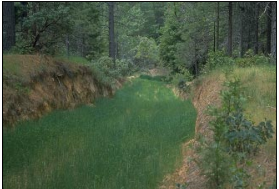
Photo 13.8 Seed and mulch (cover for seed protection and moisture retention) applied to the ground surface to promote grass growth on barren areas, closed roads, and on erosive soils.
