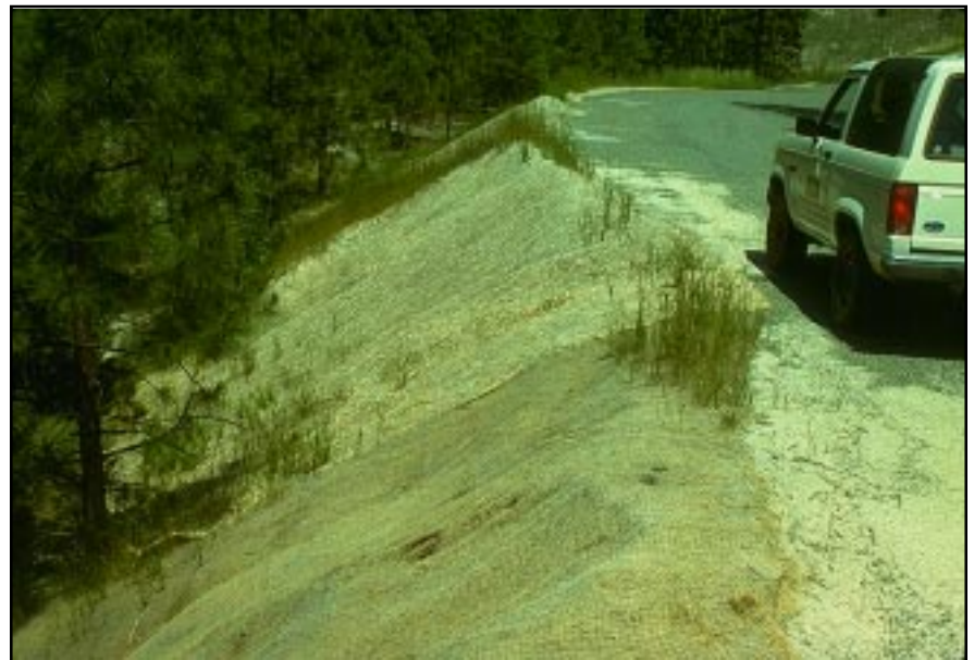
Photo 13.3 Cover fill slopes, work areas, and other exposed soil areas with straw, netting, rock, or other material to protect the ground and promote vegetative growth.
