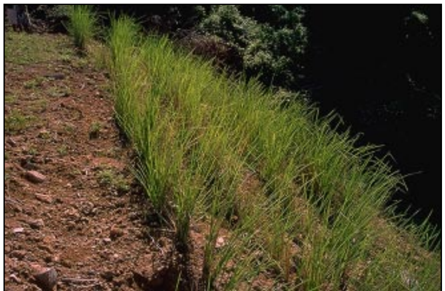
Photo 13.9 Use of Vetiver grass for slope stabilization and erosion control. Choose vegetation that is adapted to the site, has strong roots, and provides good ground cover. Ideally, use native species.
