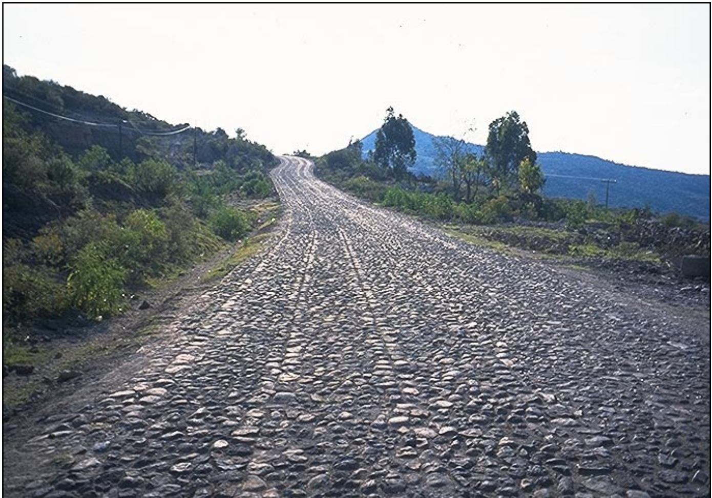
Photo 1.4 A well designed, “minimum impact” road that has an appropriate standard for its use, and a stabilized cobblestone driving surface.
