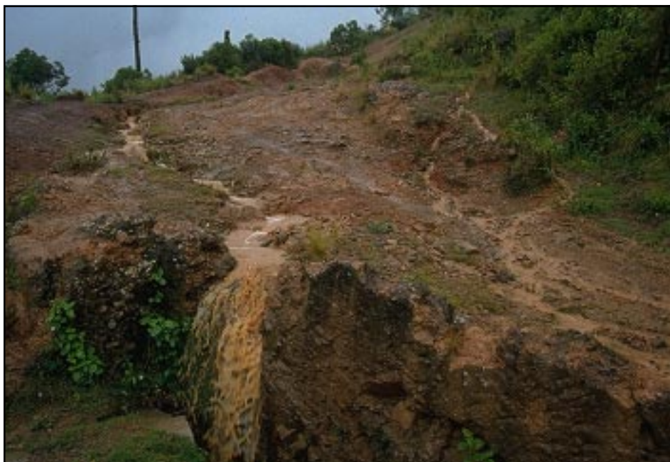
Photo 13.1 Do not leave disturbed or barren areas exposed to raindrops and runoff. Use erosion control measures to protect the area and protect water quality.
