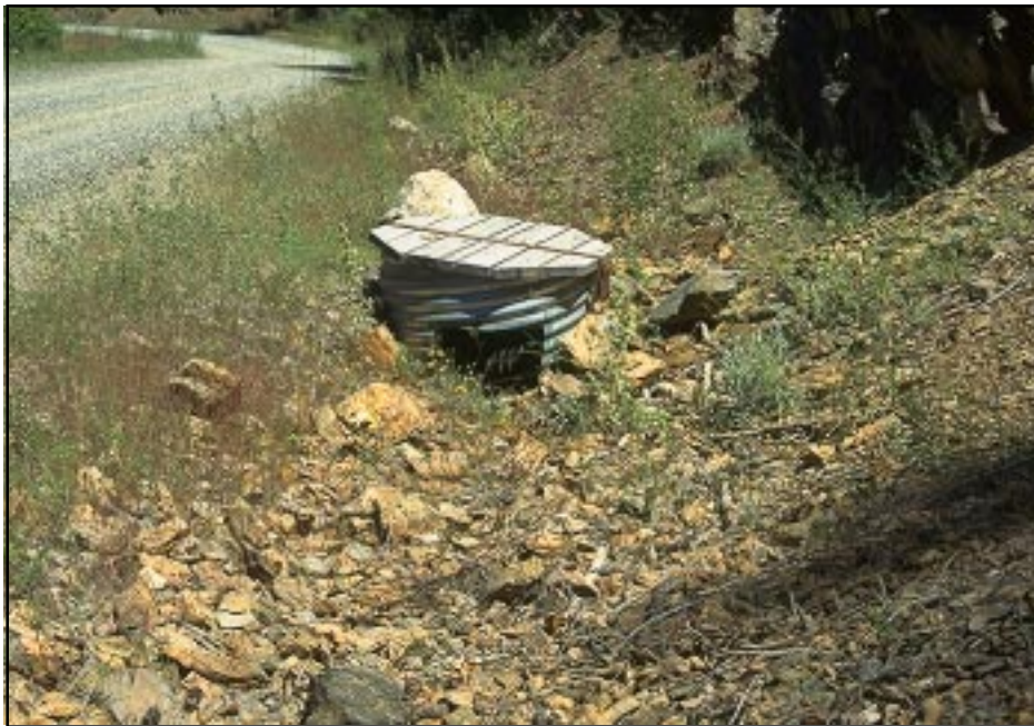
Photo 7.7 A rock armored ditch and metal drop inlet to control the water and prevent down-cutting of the ditch.
