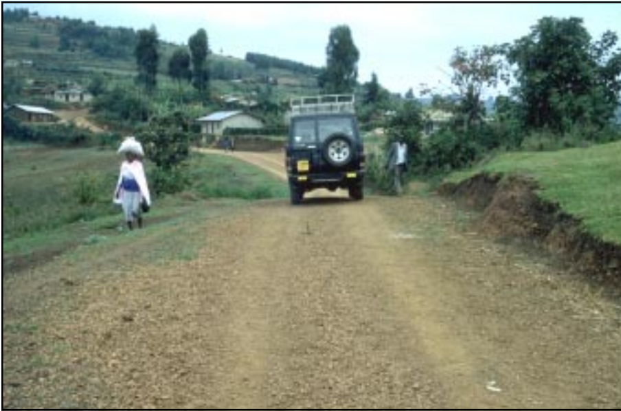
Photo 2.1 A well built road that helps serve the local population in a rural area, with minimum environmental damage.
