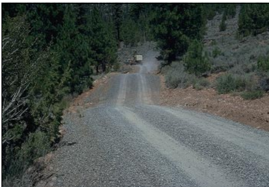
Photo 7.1 Design roads that move water rapidly off the surface of the road and minimize water concentration with the use of rolling grades and outsloped, insloped, or crowned roads.
