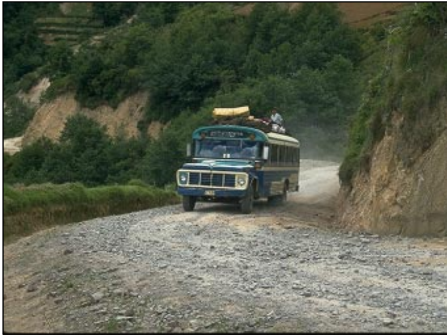
Photo 3.1 A low-volume, local road, with minimum adverse environmental impact, that serves local users by providing access between communities.
