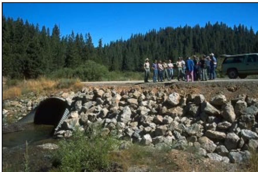
Photo 8.4 A structural plate arch pipe culvert with stream bank protection using large rock riprap placed upon a geotextile filter layer.
