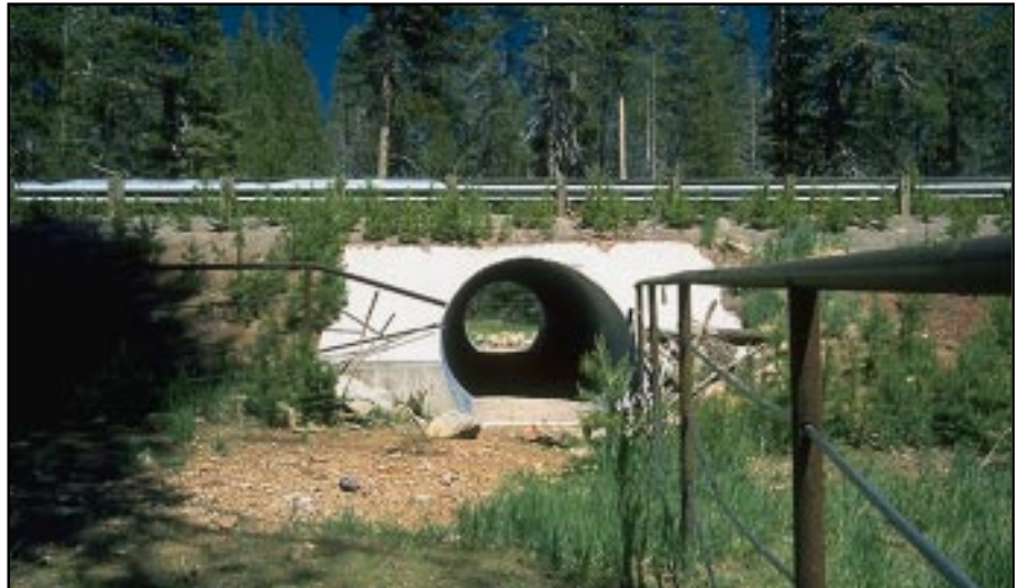
Photo 2.7 A road underpass constructed to allow animals to move safely from one side of the highway to the other.
