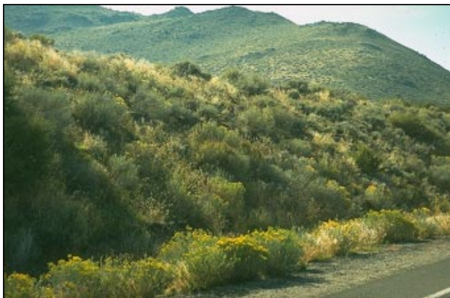
Photo 11.3 A well-stabilized cut slope, with about a 1:1 slope, that is well covered with vegetation.
