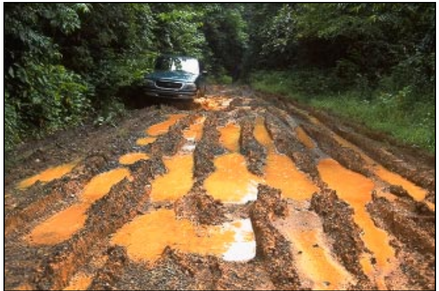
Photo 4.8 Avoid construction and other road activities during wet periods when possible. Alternatively, add drainage and surface stabilization to the roadway in weak soil areas for all-weather use.
