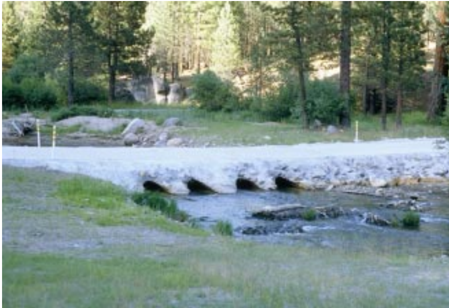
Photo 9.2 A vented ford, using multiple culvert pipes to handle low flows through the pipes, yet allow major flows and debris to overtop the entire structure.
