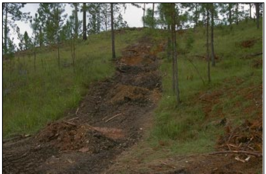
Photo 3.8 Stabilize skid roads and trails after use with water bars and apply a ground cover or other erosion control measures.
