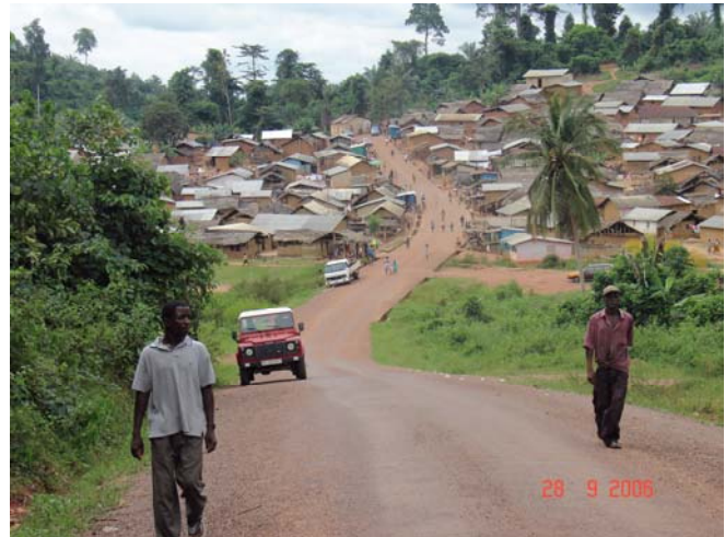
Residents of the above village in the Cape Coast area were happy that they no longer suffered from dust generation in the dry season and muddy, slippery conditions in the wet season.
