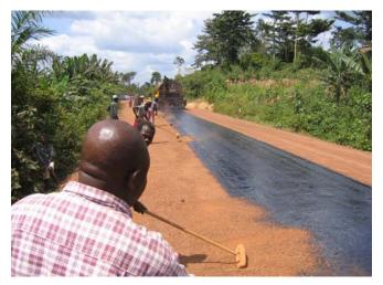
Spraying of bitumen with the use labours brooming back aggregate for the longitudinal joint immediately spraying the bitumen.
