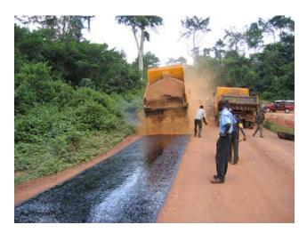
Spreading of the aggregate immediately after spraying the bitumen by the use of tail mounted chip spreaders. Notise the large amount of fines.
