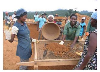
Oversize aggregate was removed by labour based methods with a good results. At a later stage a vibrating screen took over this work as seen below.
