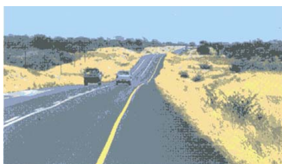
Photos 3 and 4: Gravel versus bituminous surfacing
