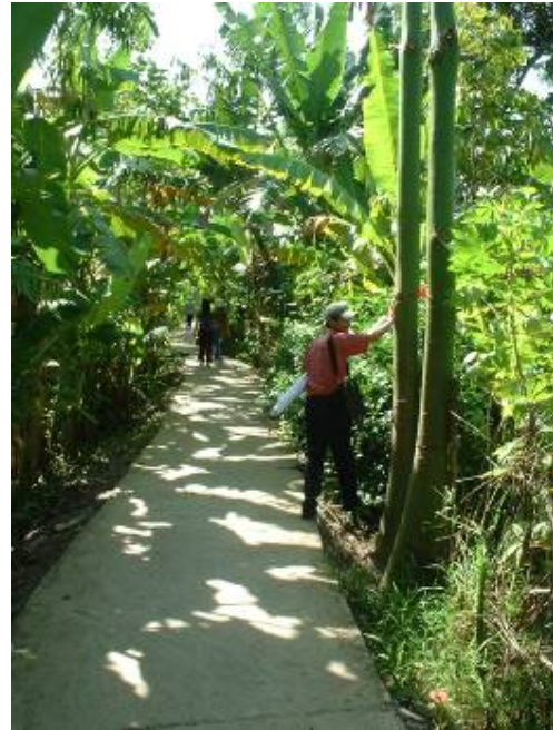
Picture 3.3: A concrete slab village road in Vinh Long province
