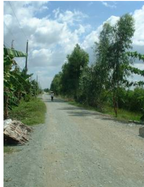
Picture 3.2: A motorable (RT2) road in Vinh Long province
