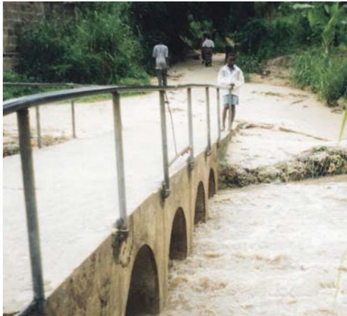
Photo 8.5-3. Repaired Yombo River bridge after heavy rains
