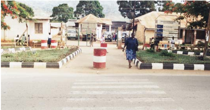
Photo 8-3-1. Entrance to the regional hospital, after the improvements
