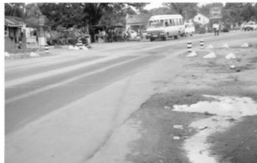
Photo 8.8-2. Example of pre-fabricated speed bump
