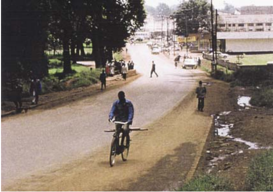
Photo 8.12-1. Kisumu road section, prior to the intervention
