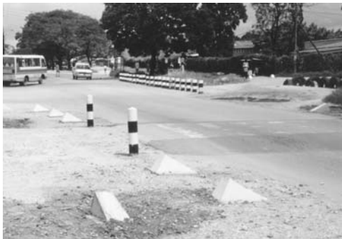
Photo 8.7-1. RZC on a collector road with a pedestrian area protected by T-blocks
