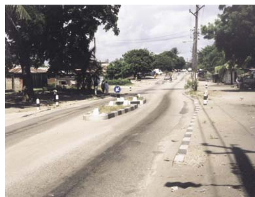
Photo 8.9-4. Overview of three crossing islands
