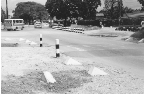
Photo 6.7. Traffic calming with RZC bollards and T-blocks separating MV and NMT
