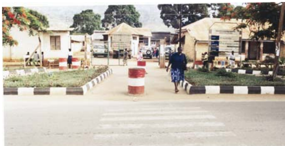
Photo 8.17-3. Entrance to the regional hospital, after the NMT improvements in 1977
