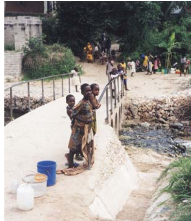
Photo 8.5-4. Yombo River bridge after the repairs
