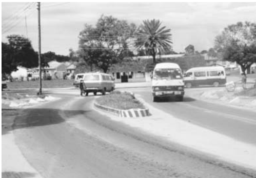
Photo 6.11. Intersection re-alignment with island
