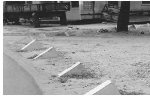
Photo 8.11-4. T-blocks separating the carriageway from the shoulder
