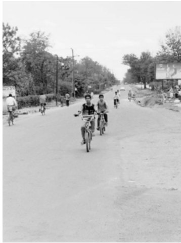
Photo 8.17-1. Old DSM Road, after widening in 1999. Wide carriageway, high speeds, lack of dedicated space for NMT, unsafe traffic conditions
