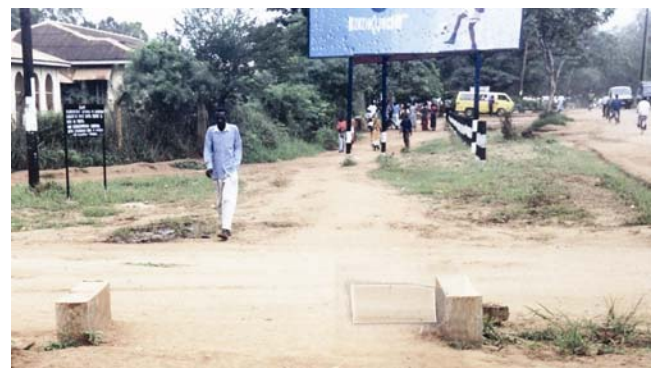
Photo 8-3-4. Pedestrians only bridge over a side drain at an intersection
