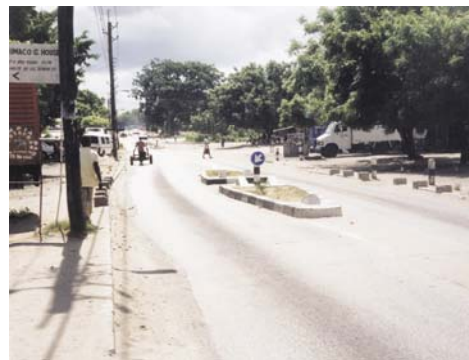
Photo 8.9-2. Pedestrian crossing island, on a collector road
