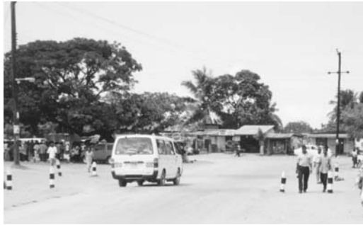
Photo 8.8-1. Two round top speed bumps at a short distance creating a safe crossing spot in DSM, similar to the ones on Nile Road
