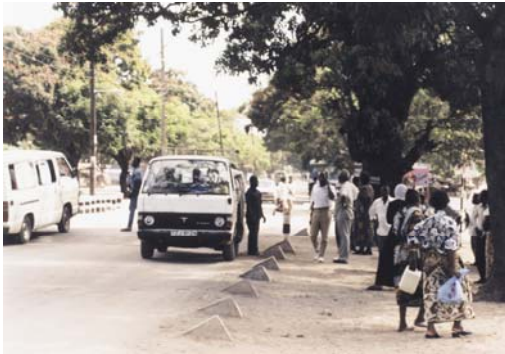
Photo 6.9. Bus-bay with T-blocks bollards separating traffic lanes
