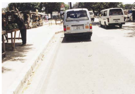
Photo 8.13.4. Same location, after the construction of the bus bays
