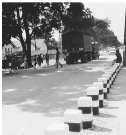
Photo 8.10-5. Carriageway and shoulder separation with bollards
