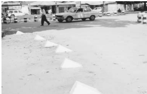
Photo 8.11-3. Shoulder of the side road separated from the carriageway
