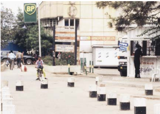
Photo 8-3-3. Walkway separated from the carriageway at the fuel station entrance
