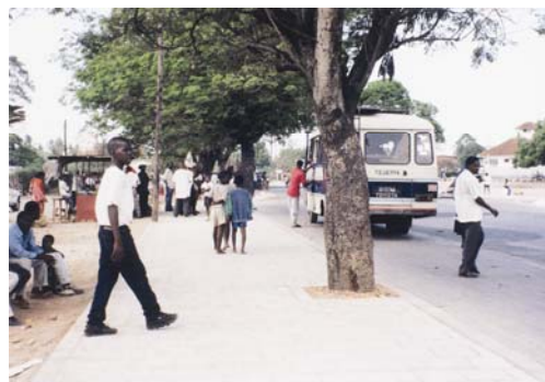
Photo 8.13.2. Same location as above, after the construction of the bus bay
