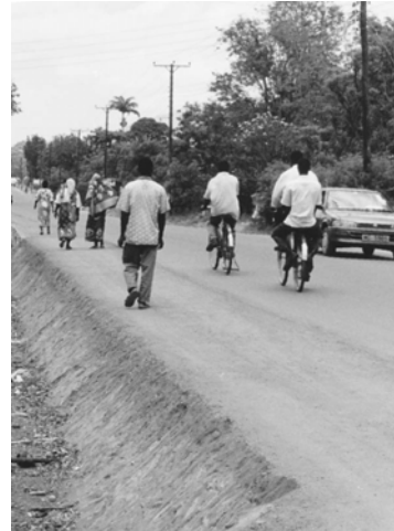
Photo 8.17-2. Old DSM Road bus bay in 1999
