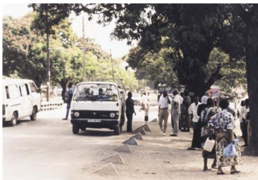
Photo 8.10-4. Effective carriageway and shoulder separation with T-blocks
