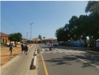
Stage 10 Construction Complete (Built Results)
