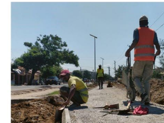
Stage 9 Support and Monitoring during Construction
