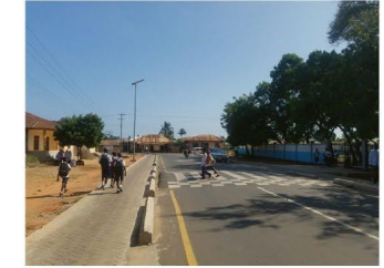
Stage 10 Construction Complete (Built Results)
