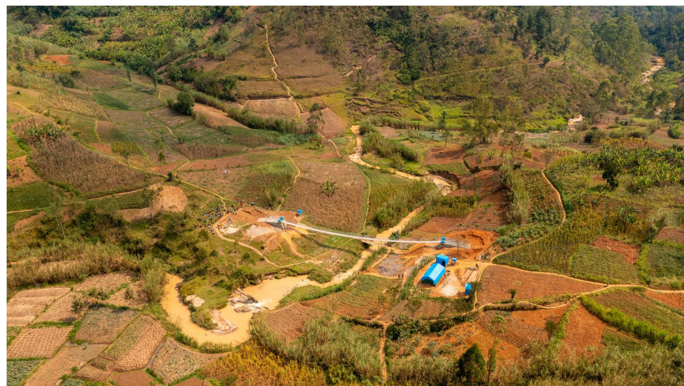
Engineered trail bridge with organic footpaths – Multi-link types
