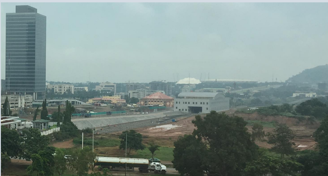
Figure 11: A Station under construction
