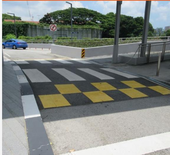
**UK, London: Road table on a local road at junction with secondary road enabling no change of level for pedestrians**
