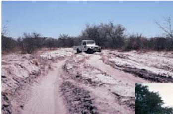
In the northern part a sand track of 45 km was upgraded to gravel road from 1980-1982 using the only available material, calcified sand. However, the road deteriorated quickly even with only 20 vehicles per day.
