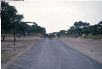
By using these materials in the pavement layers and protecting them with a bituminous surface treatment, using alluvial gravel (Otta seal) from a nearby ancient lake, the total length of 250 km were completed in the late 80-ties as seen to the right.
