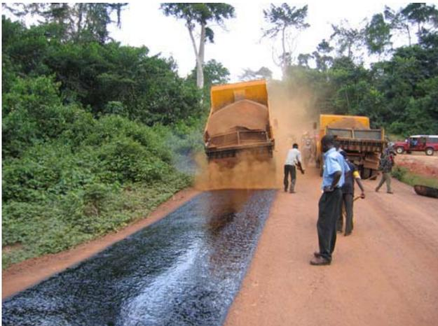
*Spreading of the aggregate immediately after spraying the bitumen by the use of tail mounted chip spreaders. Notice the large amount of fines.*
