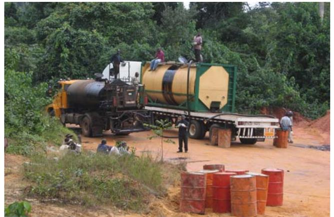
The cutting back with power paraffin to the required viscosity range was done at site.
