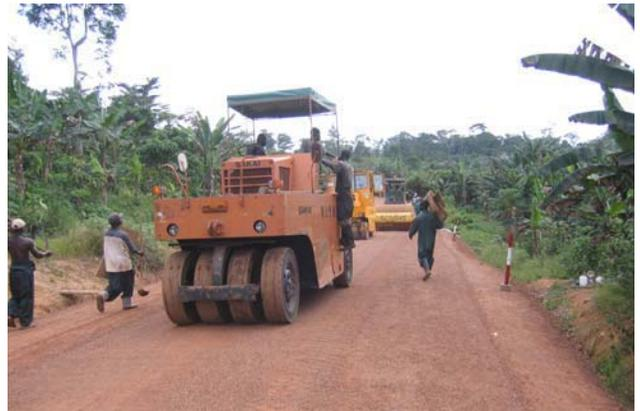
*Rolling with pneumatic rollers is an essential part of the constructing the Otta seal. It is worth to notice that an Otta seal can never be rolled too much.*
