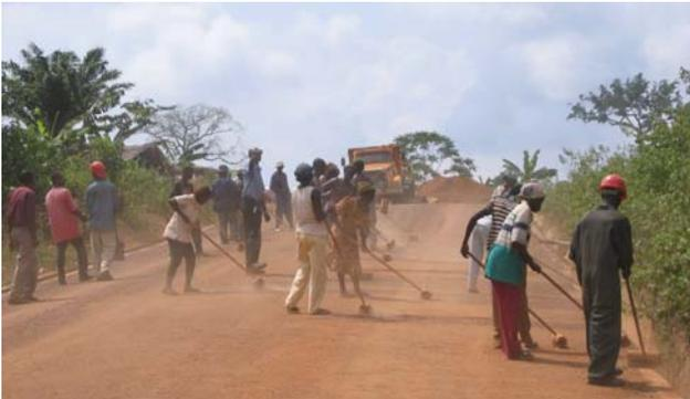
*Brooming of the base prior to sealing operations was done by the use of labours.*
