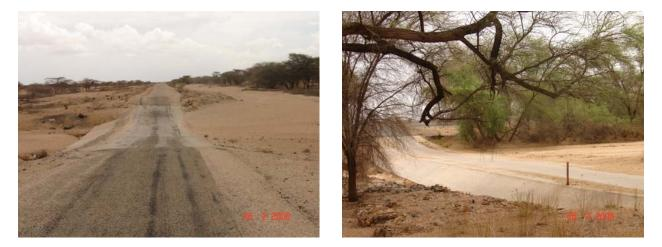
Examples of well designed drifts along the Marich Pass-Lodwar road in which the bottom of the drift, forming the road surface is exactly at the level of the river bed – a requirement for good performance.
