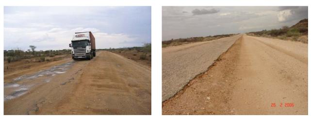
Sections of the badly deteriorated road surfacing and shoulders (left) and other sections of the same with much of the pavement structure still being intact and the graded shoulders providing an alternative roadway (right).
