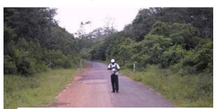
Kwale trial, "as dug" laterite as Otta Seal
