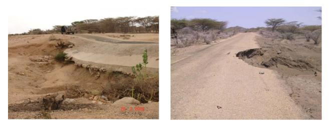
Examples of poorly designed drainage structures along the Marich Pass – Lodwar road. Insufficient depth of the downstream skirt has resulted in extensive scour of the drift (left) and a washout at a culvert outlet along the Lodwar-Kalokol road.
