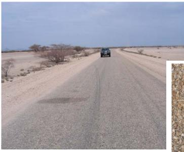
The Lodwar-Kalokol road looking towards Kalokol and showing the excellent condition of the pavement and surfacing after more than 20 years in service with practically no maintenance.
