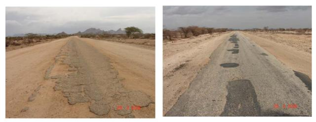
Sections of the road with no maintenance (left) and with maintenance (right) illustrating the substantial benefits of carrying out simple, routine, maintenance to extend the service life of the road.
