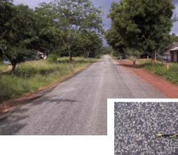
Road C 106 junction A 14. Double Otta seal using crushed coral stone.
