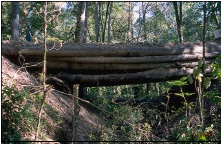
Photo 10.2 A bridge structure typically offers the best channel protection by staying out of the creek. Use local material for bridges as available, considering design life, cost, and maintenance. Inspect bridges regularly, and replace them when they are no longer structurally adequate.
