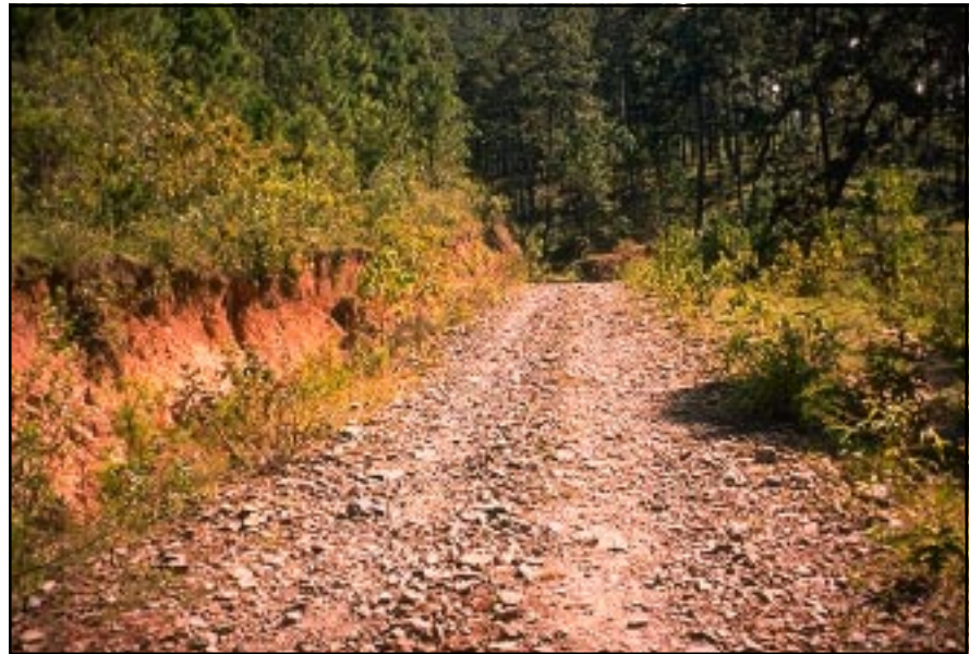
Photo 12.2 Stabilize the roadway surface with crushed rock (or other surfacing) on steep grades, in areas of soft soil, or in erosive soils.
