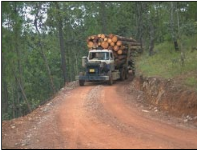
Photo 4.5 A stable logging road with aggregate surfacing. Use road surfacing materials as frequently as possible to reduce erosion and improve the roadbed structural support and rider comfort.
