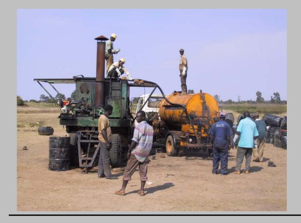
The appropriate type of binder and viscosity may be obtained by cutting back with engine oil and power paraffin on site.
