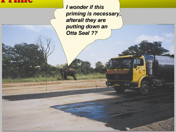
On a calcareous type of base and on stabilised bases (cement/lime) prime is required.
