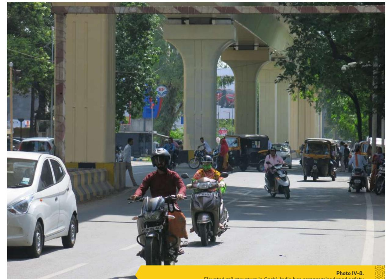
**Photo IV-8.** Elevated rail structure in Cochi, India has compromised road safety by reducing visibility and making it difficult for pedestrians to walk across the street.
